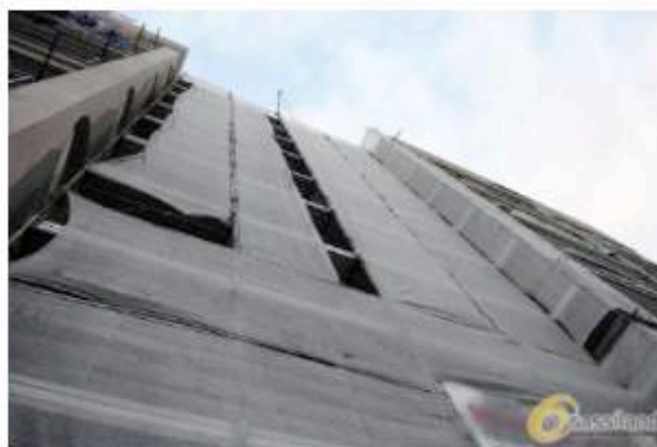
Cantiere, impalcature (foto Sassiland)
